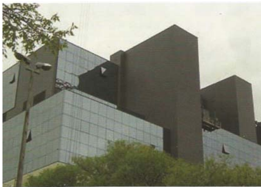
MEPAS MOSTAR – Marazzi keramičke ploče 100x100x1, 2cm, 120x60 i 60x60x1, 1cm na BWM potkonstrukciji ATK 102 Minor
