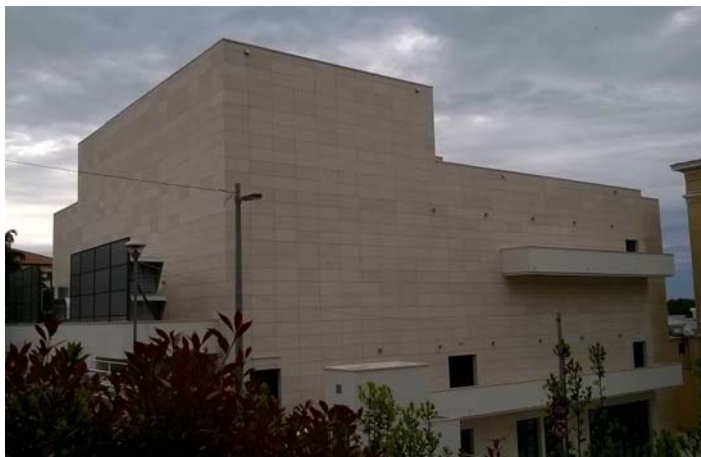
KTC Opatija 120x60x3cm kamene ploče ATK102 Minor 2000m 2
